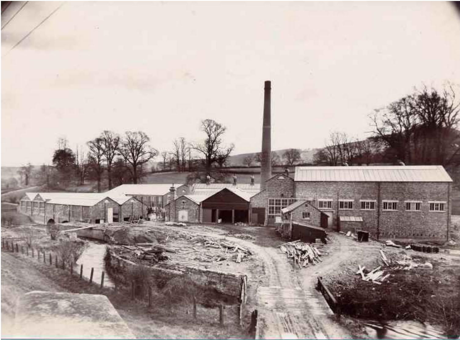
Bathford Mill - a building site in 1913
