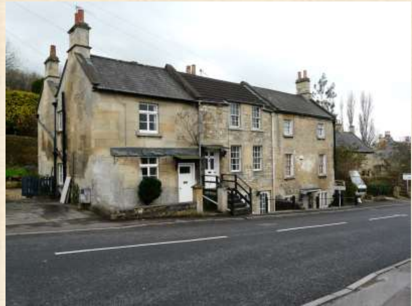
Bathford Hill houses, the two on the right, built before the mid 1700s when the road was raised to create a more even gradient so their original front doors are below the current road level.
