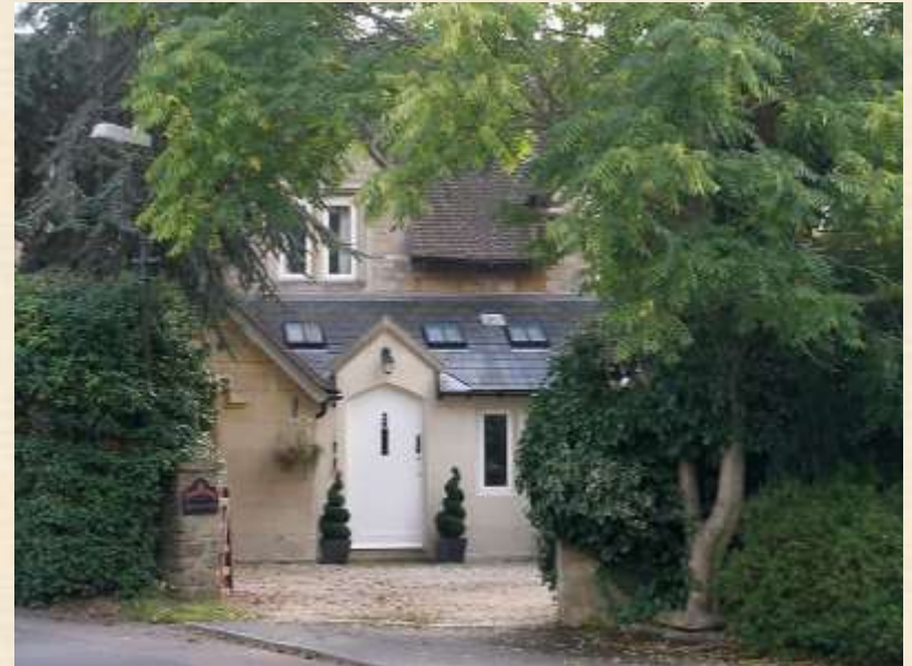
Present day, view from Church Street. Now a private residence.
