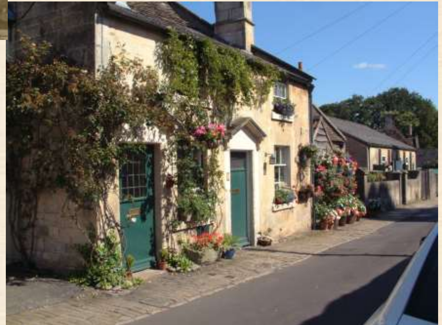
Cottages in Church Street with the well-used Parish Hall on the right
